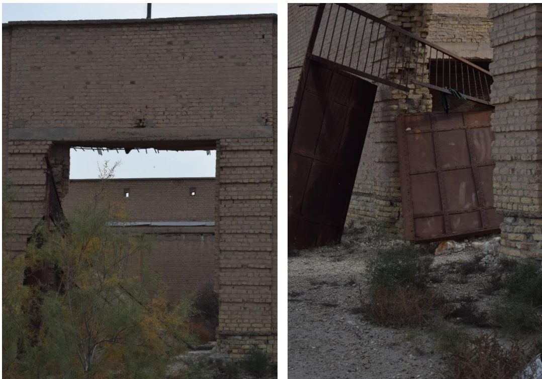
Fig. 3: Left: the only entrance to the outpost. Right: the gate (researcher)
